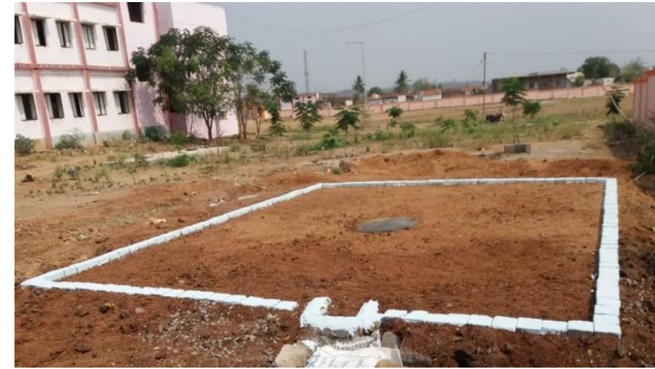
Before and after: Construction of community soak pit in water logging area
